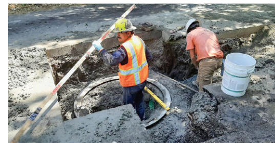
Contractor Replacing Old Brick Manhole with Concrete Manhole
