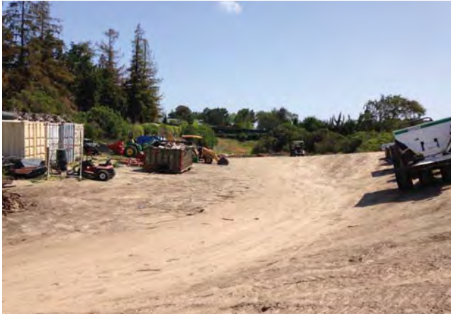
Photo 1. Proposed Water Treatment Plant (WTP) facility location.
