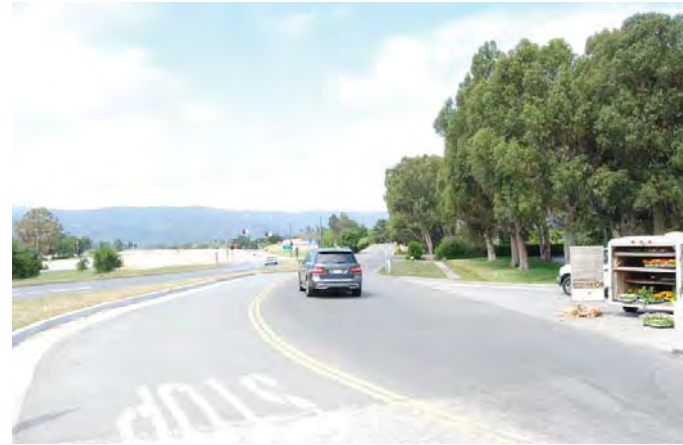
Photo 6. View looking west along the alignment on Sand Hill Road from east of golf course.
