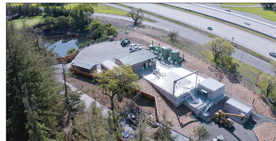
Recycled Water Treatment Plant Sharon Heights.
