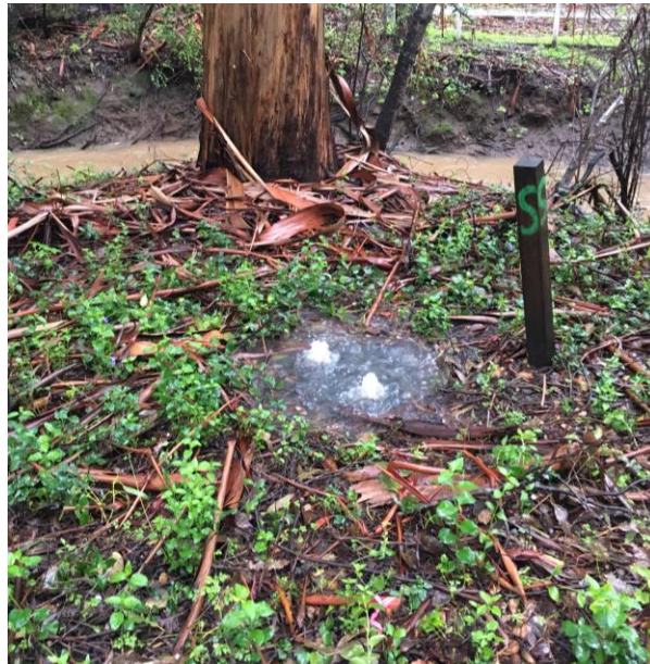
(Example of overflowing manhole)
